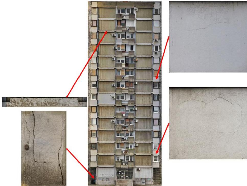
Figure 10 – Residential building – cracks and damages
