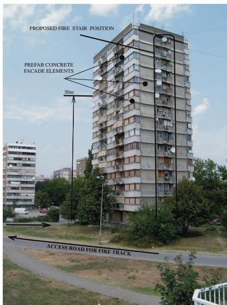
*Figure 2 – High-rise residential building with no fire stairs*
