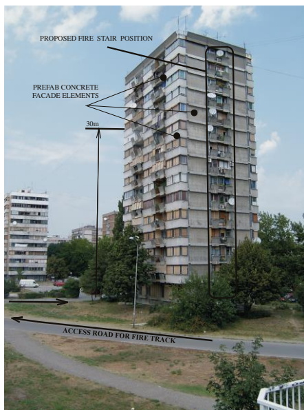
Figure 2 – High-rise residential building with no fire stairs
