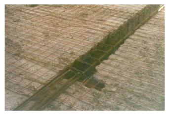
Figure 27. The wire-mesh reinforcement in the slab
