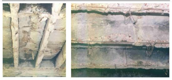
Figure 8 and 9. The characteristic view of the pan-joist structure after fire
