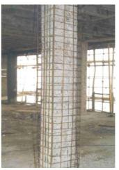
Figure 12. The placing of the new column reinforcement
