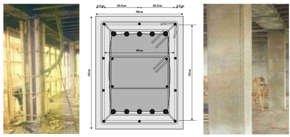
Fig 14. Placing of the new layer on the column
