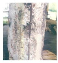
Figure 6. Typical view of the column after fire
