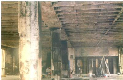
Figure 5. The view of the damaged structure on the 8th floor after the fire and clearing
