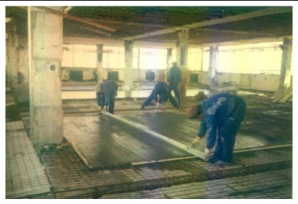
Figure 28. Concreting of the new slab
