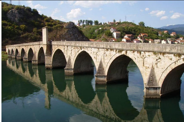
Figure 11 – Mehmed Paša Sokolović Bridge: view of the bridge during the last reconstruction [12]
