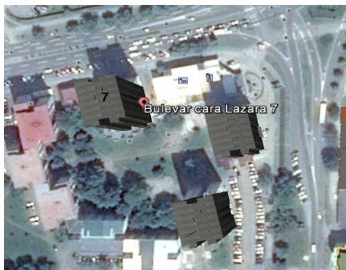
Figure 6 - Position of the building 3
