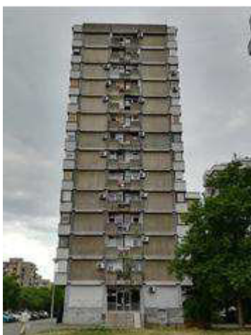
Figure 1 – Case study building elevation
