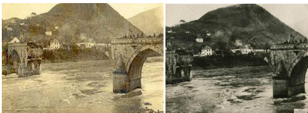
Figure 10 – Mehmed Paša Sokolović Bridge: view of the demolished arches in 1915 [12]
