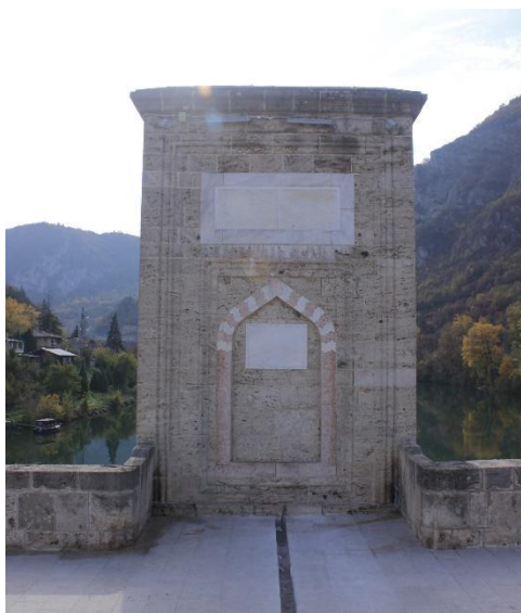
Figure 12 – Mehmed Paša Sokolović Bridge: view of the central pile after the last reconstruction [12]
