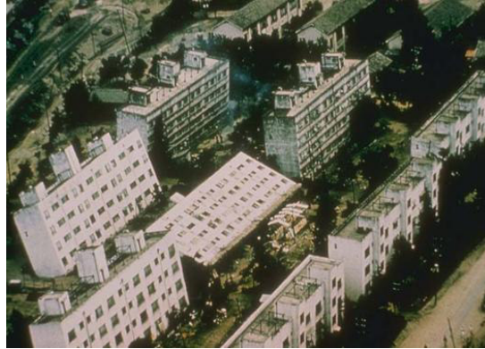
Figure 1 – Geohazard caused by liquefaction [9]
