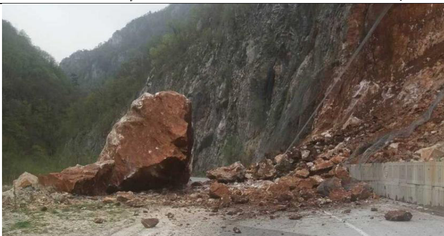
Figure 2 – Rock slide as a form of a sliding process. Very often such hazards are defined as landslides even though there is a significant difference in the mass transfer mechanism. Because of this, defining hazards in sliding processes is very important for adequate prevention. [6]
