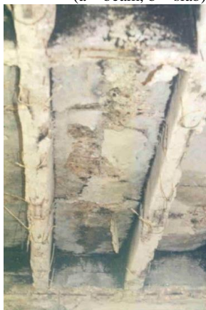
Figure 17. Influence of defects on fire damages degree in pan joist floor system
