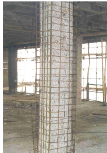
Figure 12 and 13. The placing of the new column reinforcement
