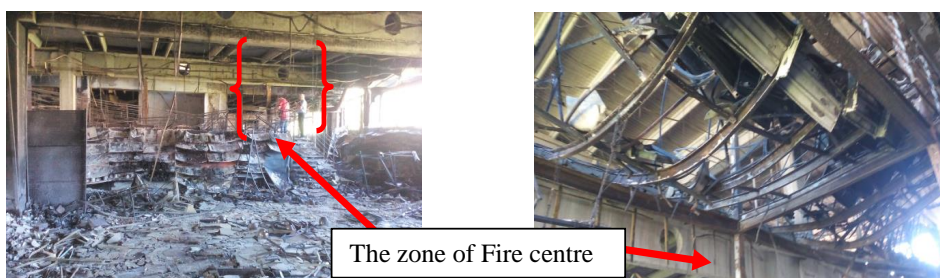
Figure 7. The zone of fire centre – observed from the Hall 2 basement
