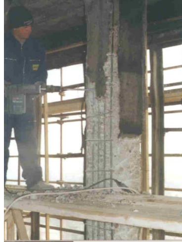
Figure 10 and 11. Removal of the damaged concrete layer from the column
