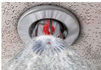
Figure 29. Sprinkler head ( https://www.houseidea.pw )
