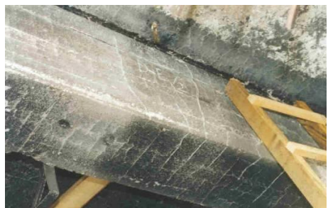
Figure 6. Cracking – mesh like cracks
