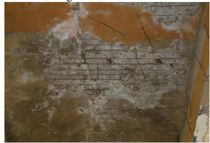
Figure 4. Sloughing off spalling (slab)
