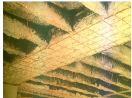
Figure 17 and 18. Removal of the damaged concrete cover and drilling a slab opening
