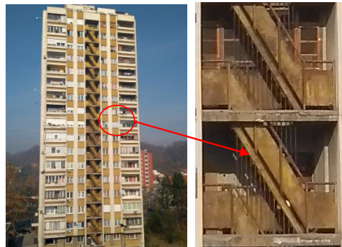
Figure 45. Consequences of poor maintenance of an external fire escape stairway (high-rise building Tuzla, B&H)
