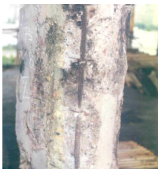
Figure 6. Typical view of the column after fire
