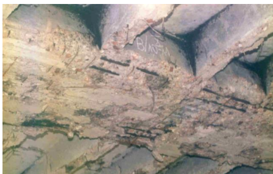
Figure 7. The characteristic view of the longitudinal beam after fire
