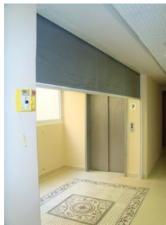
Figure 13. Fire curtains for elevators
