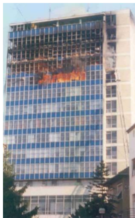
Figure 16. Spreading of fire in both vertical directions [9]
