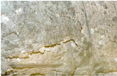
Figure 3. Sloughing off spalling (beam)
