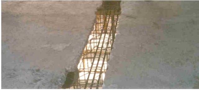
Figure 26. The reinforcement of the new beam
