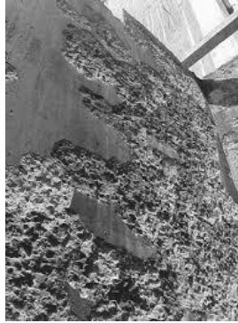
Figure 4. Spalling in concrete [1]
