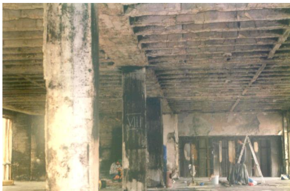
Figure 5. The view of the damaged structure on the 8th floor after the fire and clearing
