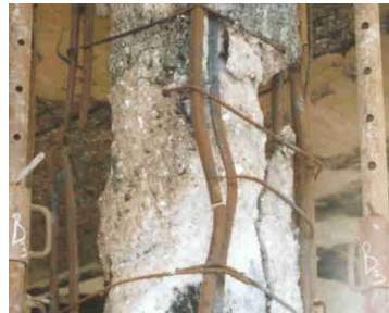
Figure 8. Plastic deformations and breaking off of bars
