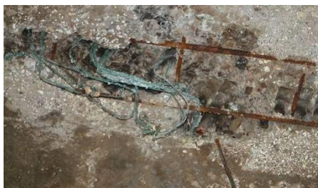
Figure 15. Local deep overheating of concrete and deformed rebar due to wirings within cross-section (a – beam, b – slab)
