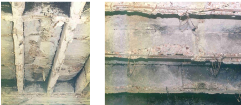
Figure 8 and 9. The characteristic view of the pan-joint structure after fire
