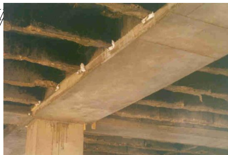
Figure 20. View of the new protective cover on the down part of the beam
