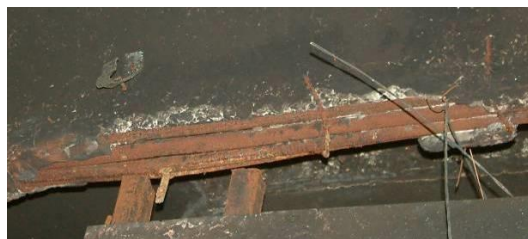
Figure 14. Characteristic damages of improper reinforced rib due to fire
