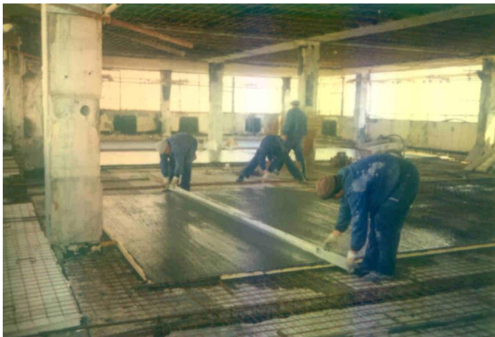
Figure 28. Concreting of the new slab
