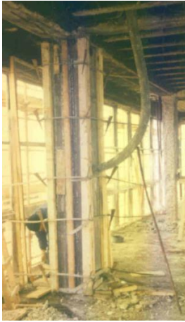
Figure 14. Placing of the new layer on the column
