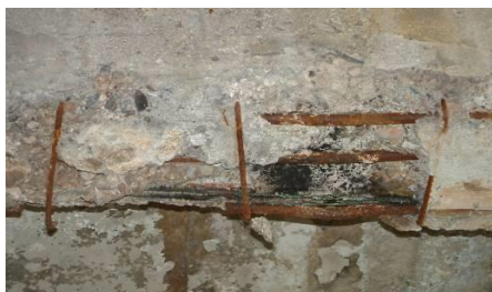
Figure 15. Local deep overheating of concrete and deformed rebar due to wirings within cross-section (a – beam, b – slab)
