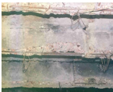
Figure 13. Typical damages of pan joist floor system due to fire
