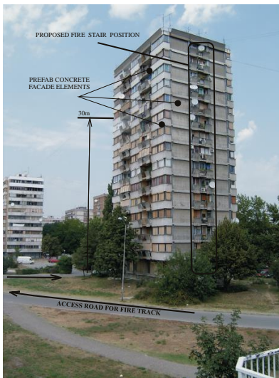
Figure 2. High-rise residential building with no fire stairs
