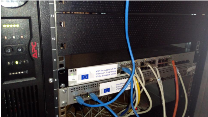
18. D-link DGS-1210-28 network switch (1 piece) and MikroTik RB2011UIAS VPN router (1 piece)
