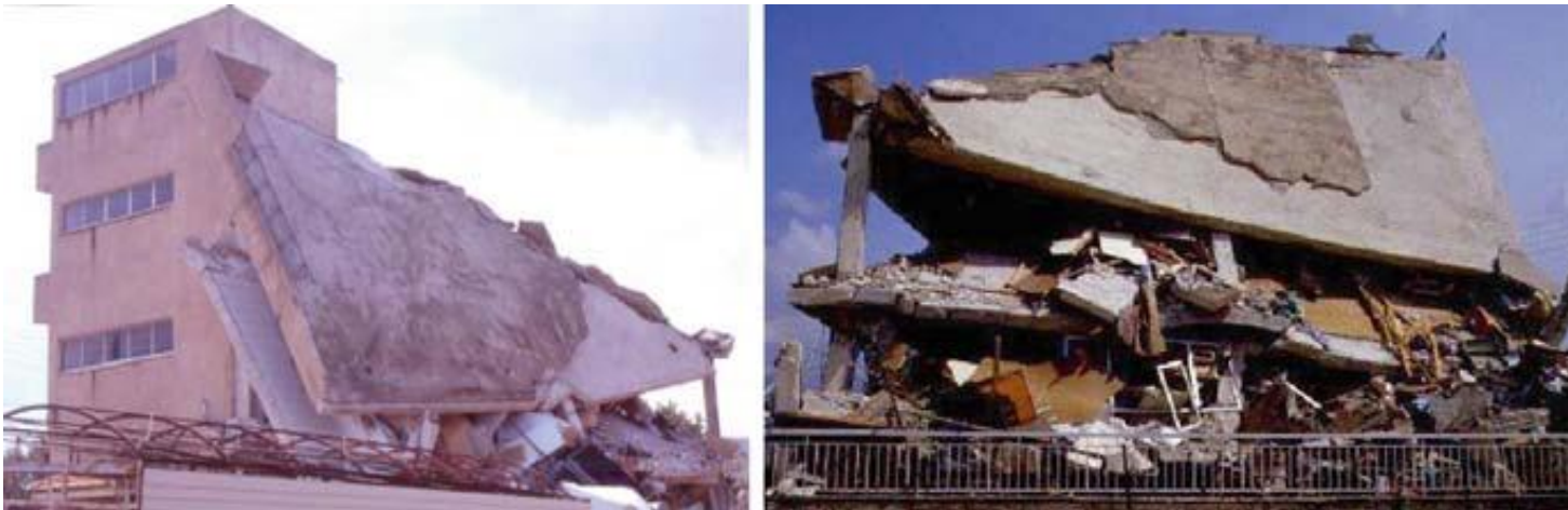
Collapse of a building due to torsional response, Athens (1999) earthquake
