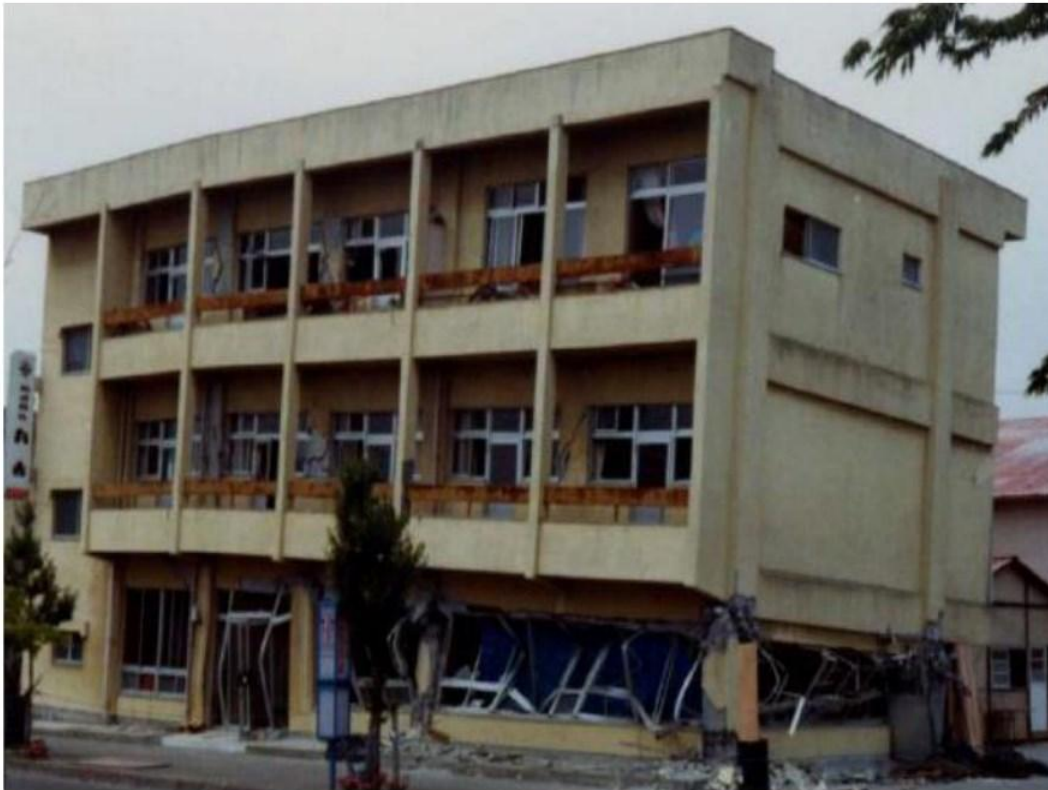
Damage of three storey building during 1978 Mijagi-Ken-Oki earthquake
