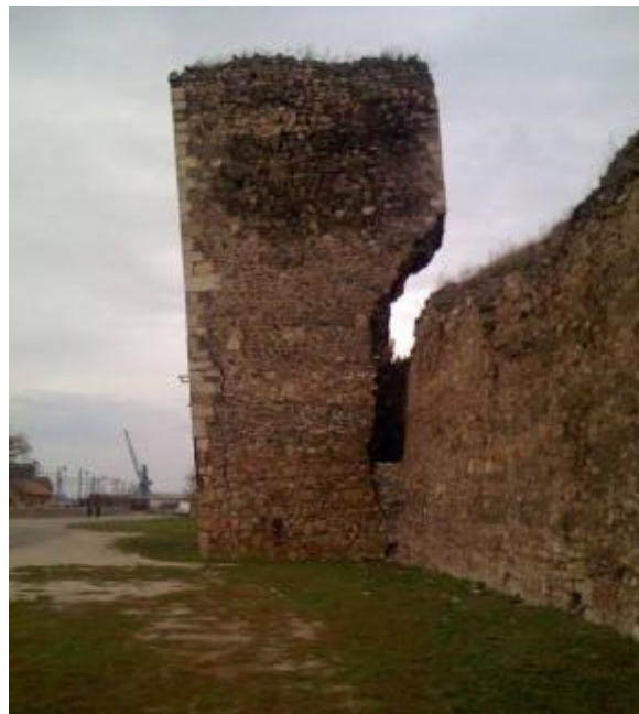
Fig. 4. Rotation (tilting) of Tower 11
