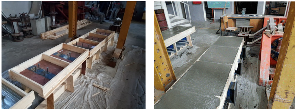
Fig. 5. Casting of the concrete
