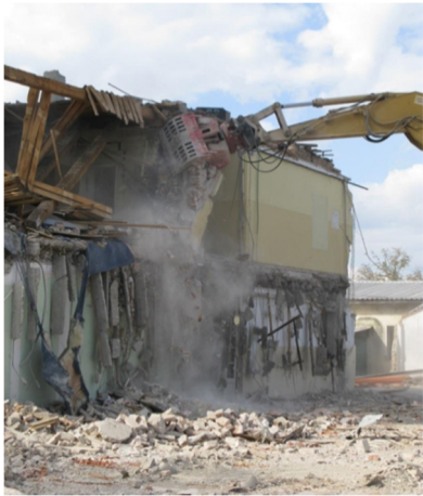
Fig. 4. Demolition of the TMD building
