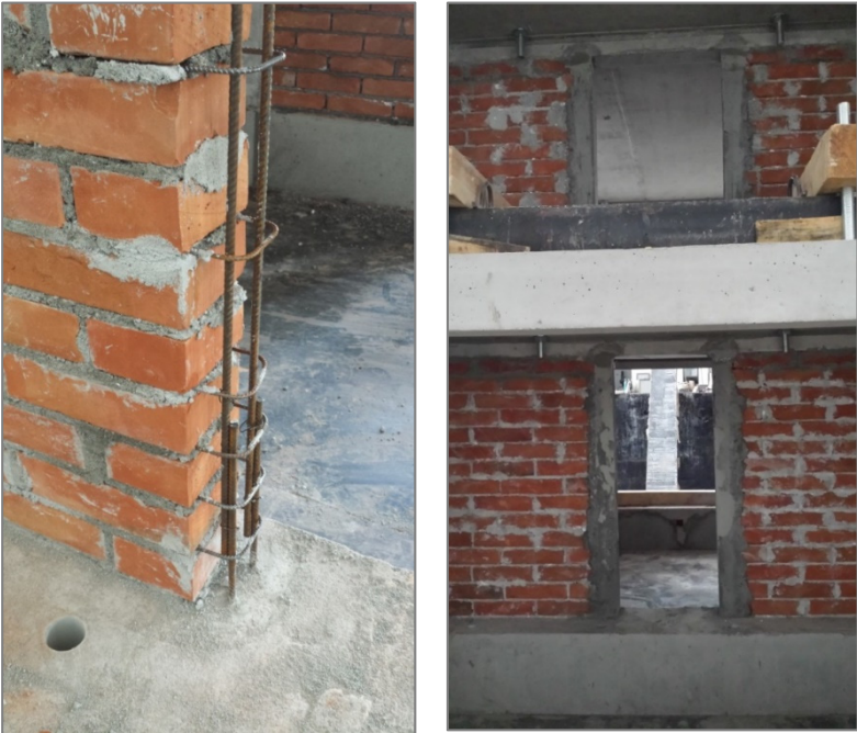
Fig.5 Construction of MODEL 2 – insertion of infill and RC vertical ties
