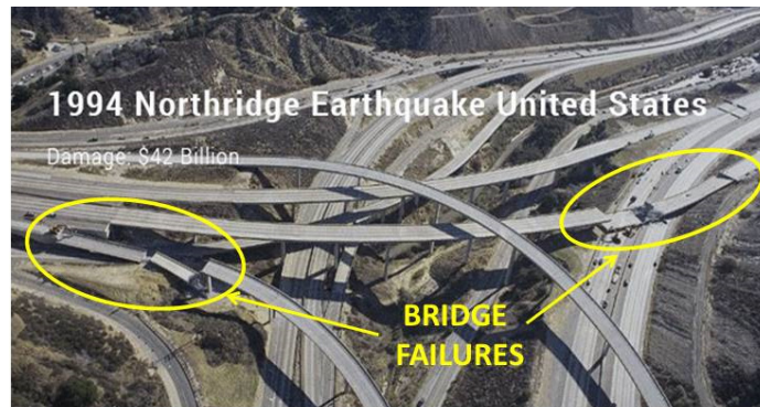
Fig. 5. Two bridge failures on I-5–State Road 14 Interchange
