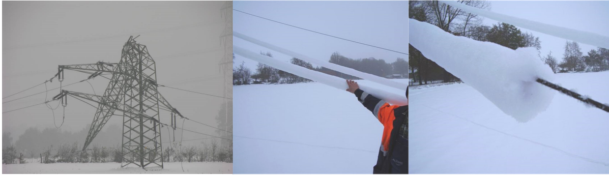
Fig. 11. Collapsed mast of transmission line (left) and rough ice agglomeration at transmission cable (center and right) after the atmospheric icing event at November, 25th, 2005
