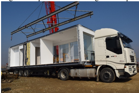
Fig. 22. Loading of finished modules
