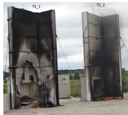
Fig. 13. 57 min from the start – wood crib has burned up
