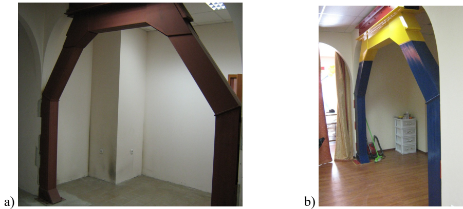
Fig.4a,b. Steel-frame system developed for strengthening of reinforced concrete frames with infills, as well as to masonry structures
