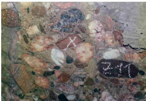
Fig. 3. Aggregate spalling
