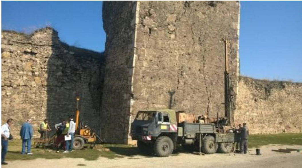
Fig. 6. In-situ investigation of Tower 11 foundation soil (left: CPT, right: borehole drilling)
