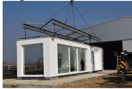
Fig. 21. Preparation for loading for transport
