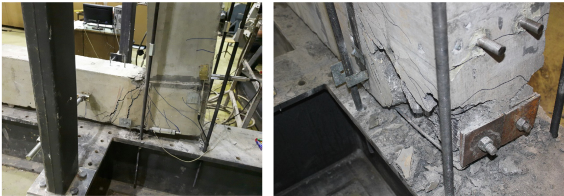
a) failure state of a specimen S1, V.D. b) failure state of a specimen S5, H.D.
