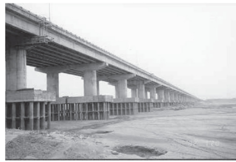
Fig. 7b. Xizhou bridge (January, 2002) (Wu et al. 2002)
