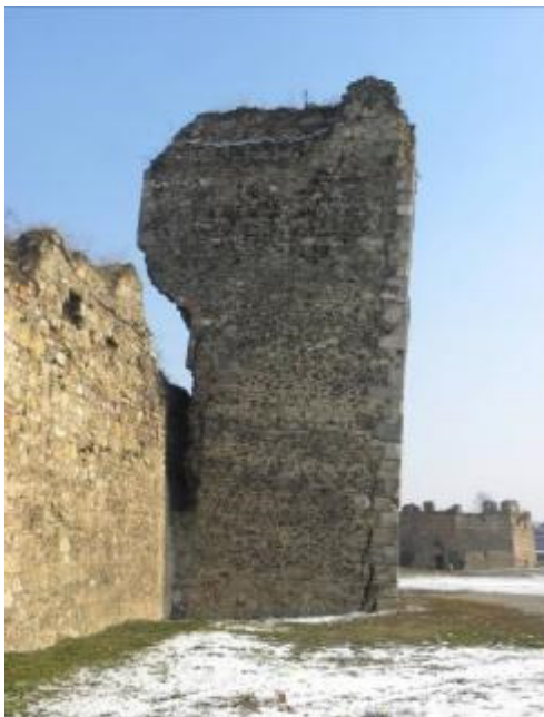
Fig. 4. Rotation (tilting) of Tower 11
