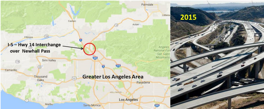
Fig. 1. Interstate I-5 and State Road 14 Interchange over the Newhall Pass
