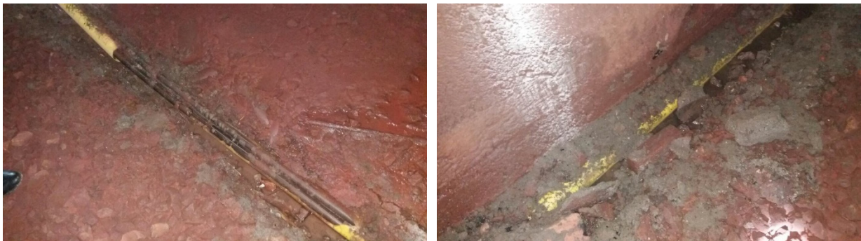
Fig. 4. Telecommunication cables before start of works
