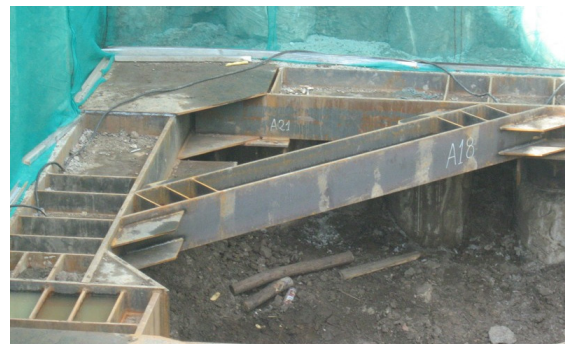
Fig.4b. Hunch box shape element section
