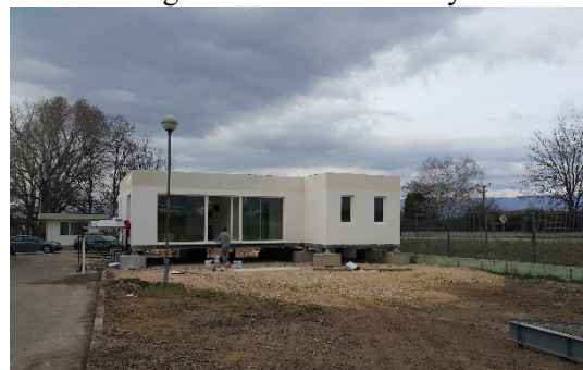
Fig. 25. Finalizing on-site works
