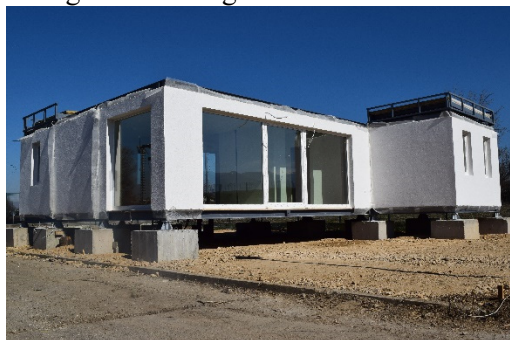
Fig. 24. Leveling and roof installation
