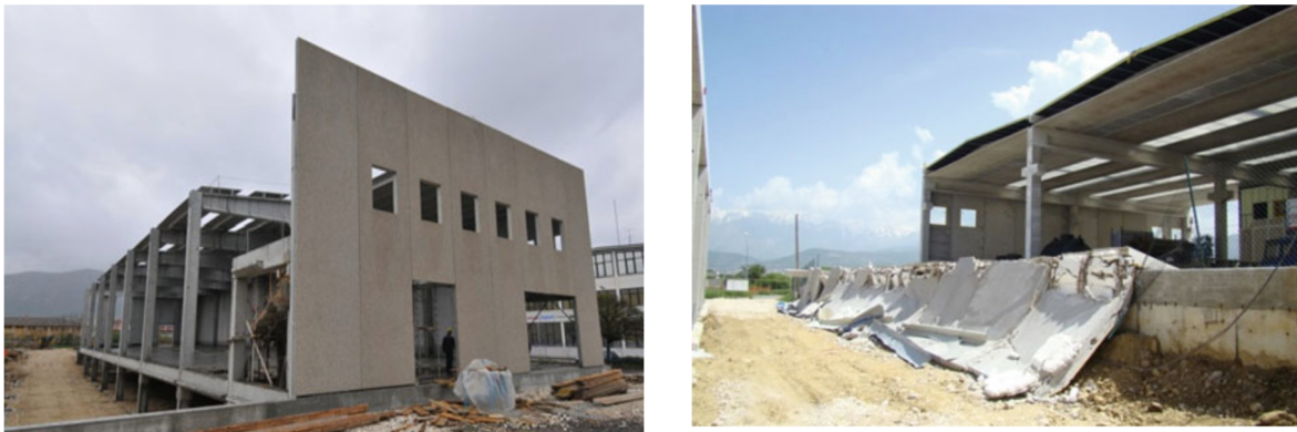
Fig.2 Evidence of good and poor behaviour during recent Italian earthquakes (M. Fischinger et al., 2014 – left; Toniolo and Colombo, 2012- right)
