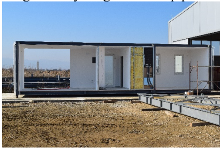
Fig. 20. Preparation for loading for transport
