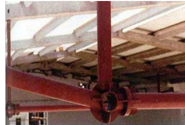
Fig. 24 Detail of joint in bottom chord
