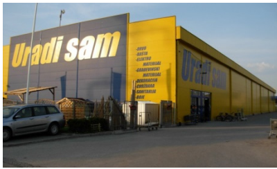
Fig. 21. View of the hall before the fire
