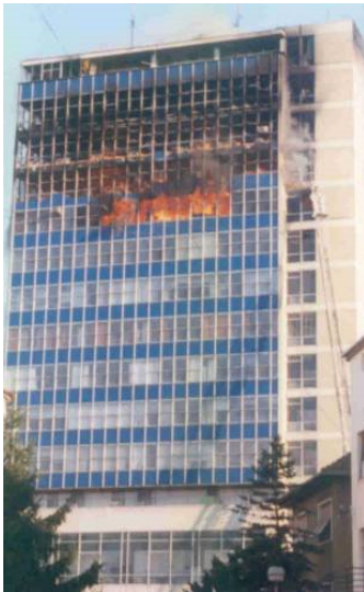
Fig. 18. Spreading of fire in both vertical directions
