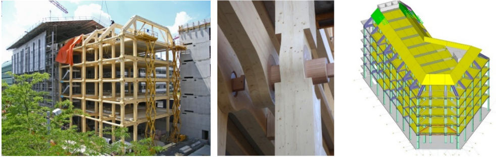
Fig. 8. Tamedia office building, Switzerland
