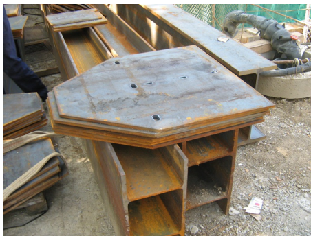
Fig.4a. Steel plate with elliptical holes
