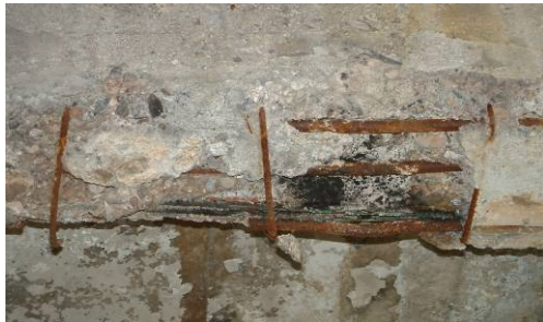
Fig. 17. Local deep overheating of concrete and deformed rebars due to wirings within cross-section (a – beam, b – slab)
